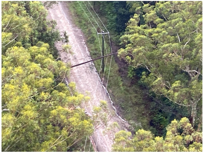
Figure 10 Vegetation near the network can cause failures and fires
