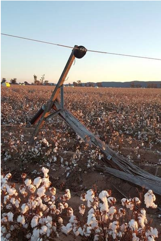
Figure 8 Pole failure in a cotton field
