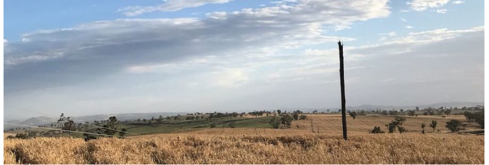
Figure 5 Electricity network damage due to high winds, Young, December 2020
