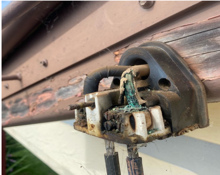
Figure 12 High impedance neutral identified through the trial
