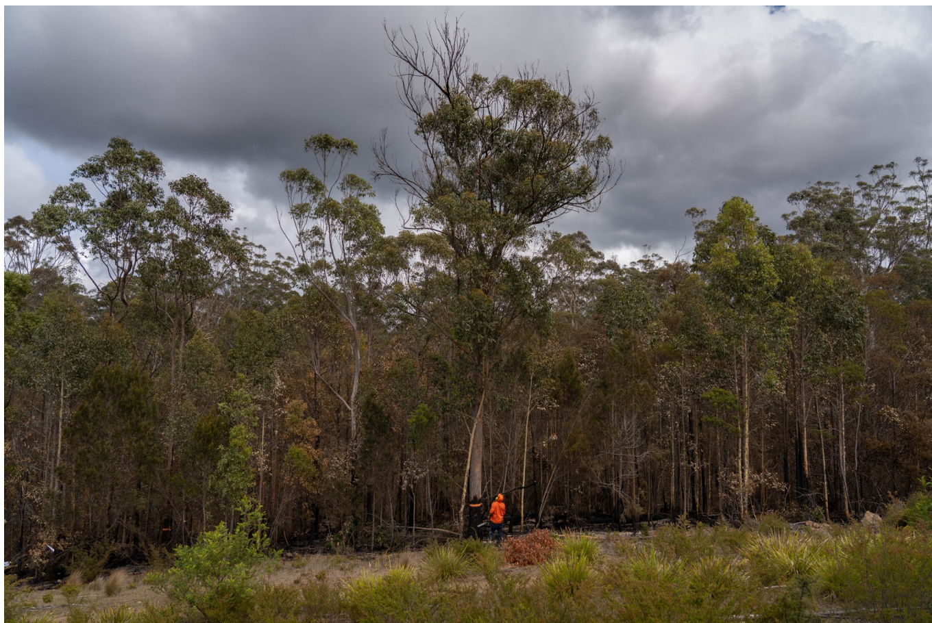
Figure 21 Treatment of bushfire affected hazard trees adjacent to an electricity easement
