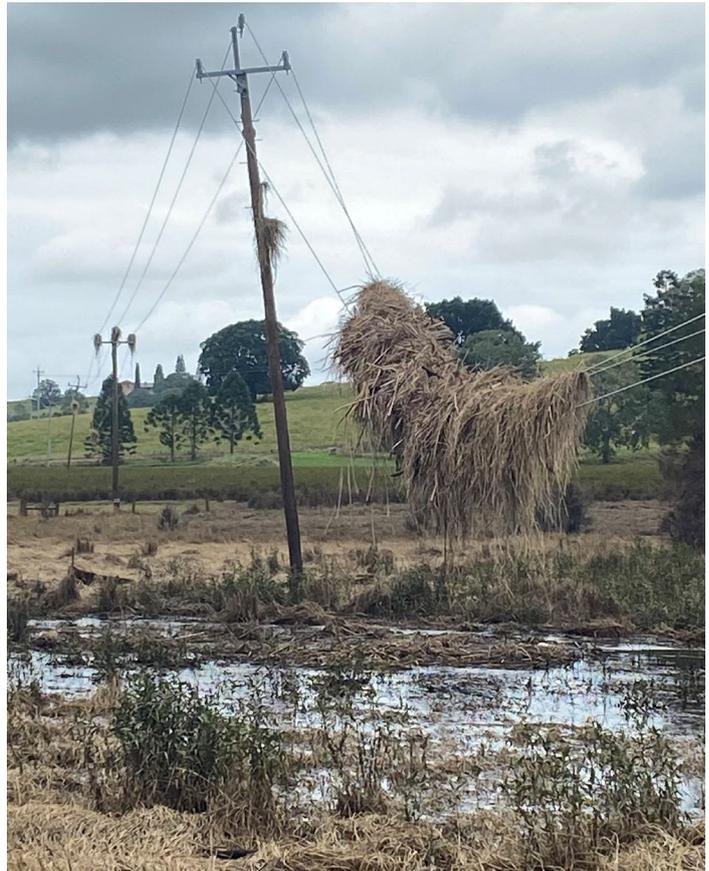
Figure 8 Essential Energy network damaged by floodwaters
