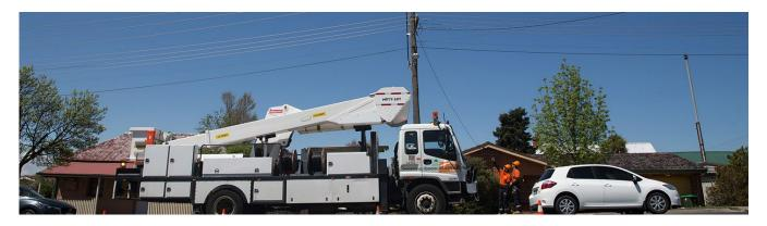
Figure 9 Essential Energy workers preparing to replace an overhead service main
