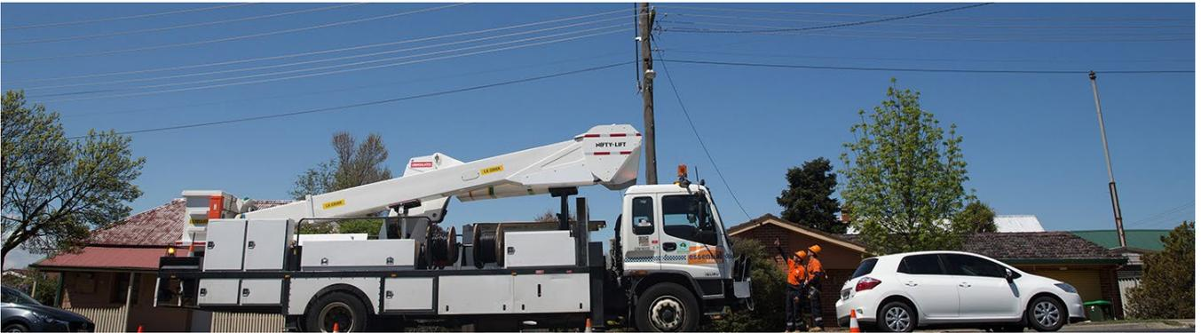
Figure 9 Essential Energy workers preparing to replace an overhead service main
