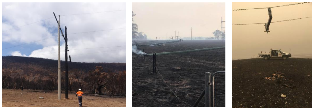
Figure 7 - Left : Timber vs Composite after bushfires , Middle: Timber CCA poles 2019/20 bushfires , Right : Timber pole burnt away, only composite cross arm remaining
