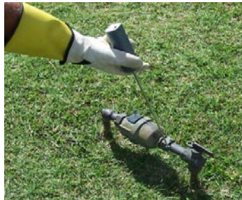
Detection of stray voltage
