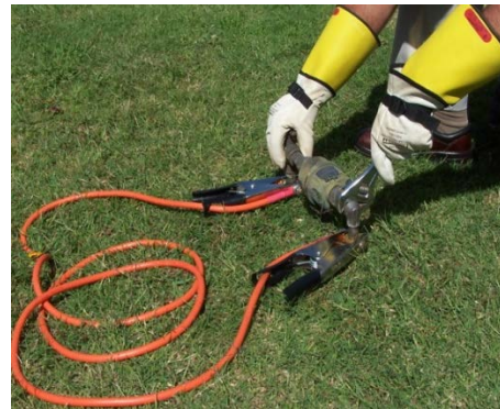
Bridging out of water meter
