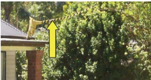
Insulated matting and tiger tail fitted to overhead service line
